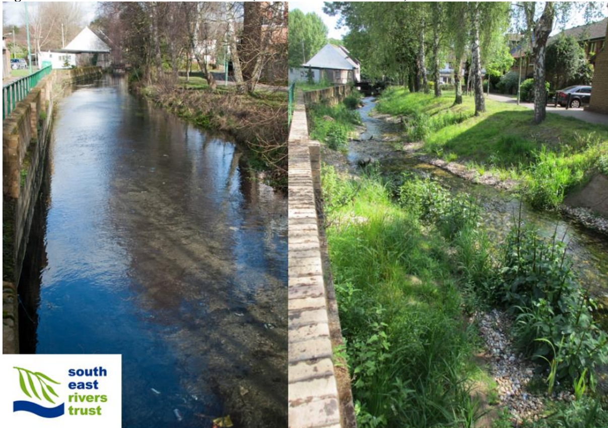
Figure 4 - Restoration works at Butter Hill (©South East Rivers Trust)
