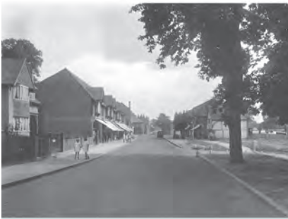
Malden Road before road widening
