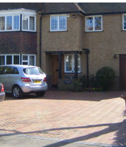
Front garden replaced with paving
