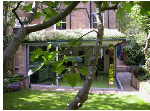
Figure 14: An extension and a sunroom. Designed with an eco-friendly green roof system to address the need for more space. Courtesy of Cullinan & Buck Architects.
