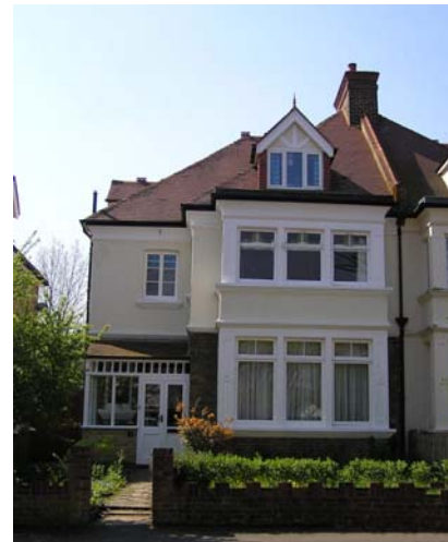
Figure 27: The Edwardian dormers are 'original' and sit comfortably within the roofscape
