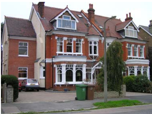
Figure 10: Original joinery appropriate for the period of dwelling and opening.
