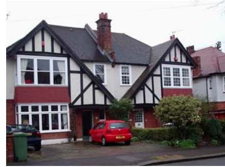
Figure 11a: Original windows to the left property are retained but not to its partner.
