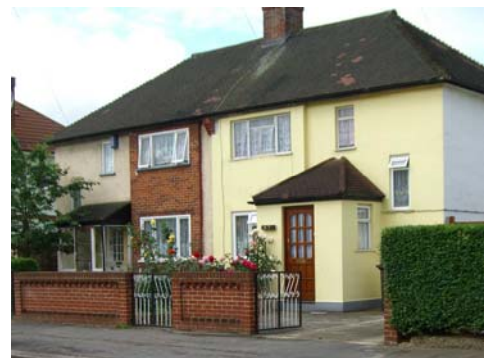
Figure 23a: Two differently styled porches, which bear no regard for the original building style.
