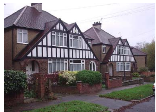
Figure 1c: Typical 1920's suburban semi-detached dwellings.
