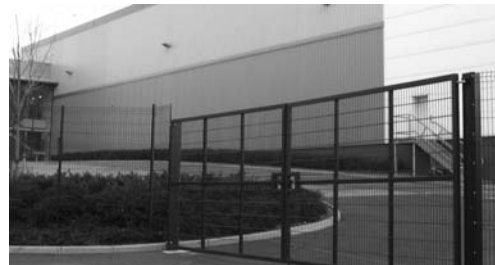
▲ A secure physical barrier to industrial units
