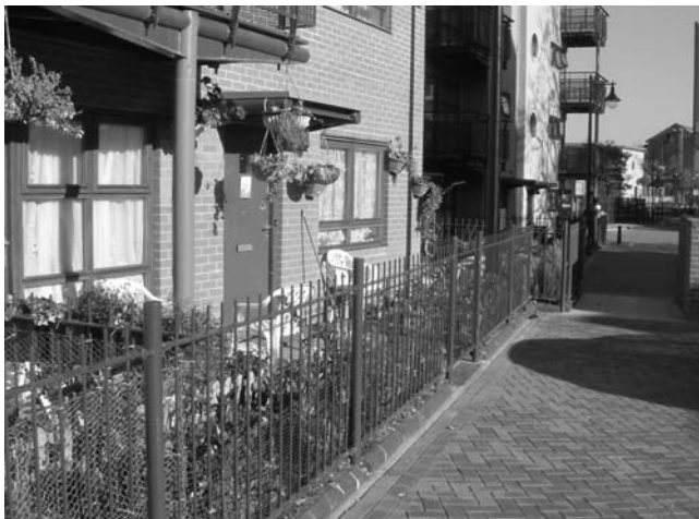
◀ A high standard of design and materials with adequate security creates a safer and more attractive environment
