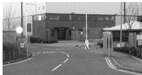
▲ A manned gatehouse is advisable for larger industrial developments
