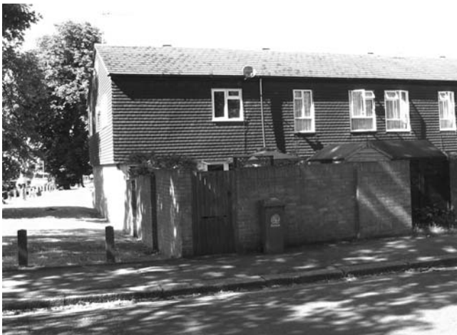
◀ Obscured views to and from the street and the presence of potential climbing aids create ideal conditions for potential intruders
