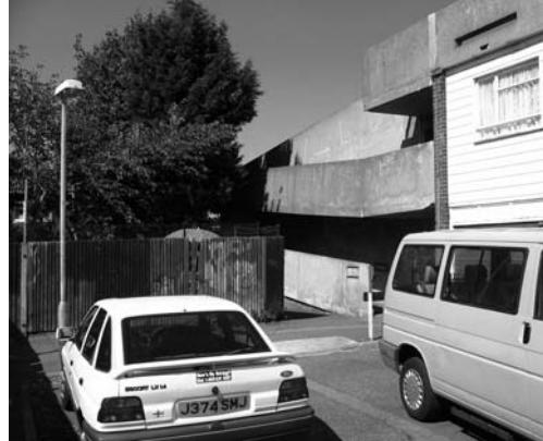
▲ Obscured access routes, such as this walkway, can lead to under-used, isolated and unsafe environments
