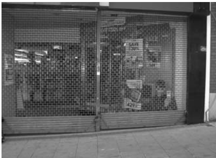
▲▲ External open grille shutters are preferable to solid roller shutters
