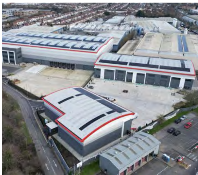
In recent years lots of sites in Beddington SIL have come forward for redevelopment, providing new and modern industrial premises that meet modern needs. This image shows a recent development on Redhouse Road.
