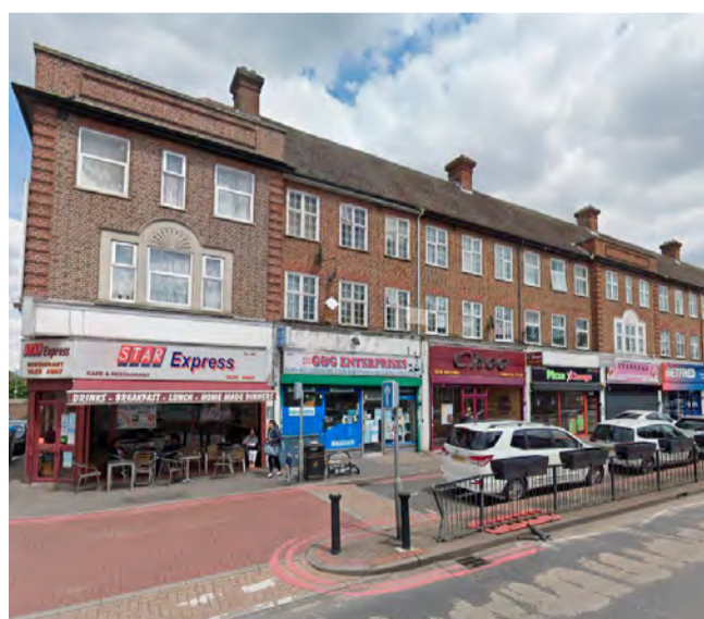
Rosehill District centre is three storeys buildings that are consistent with the character of wider St Helier.
