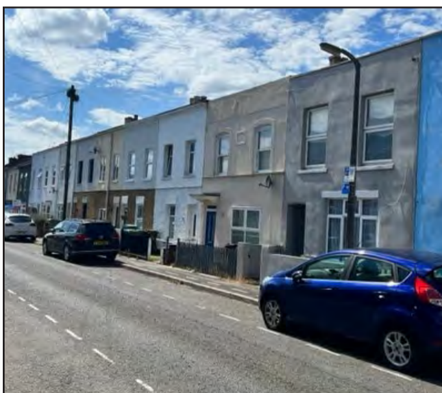
Parts of the neighbourhood have formal heritage recognition. Longfellow Road ASLC, located in Worcester Park, has examples of good Victorian terraced homes.
