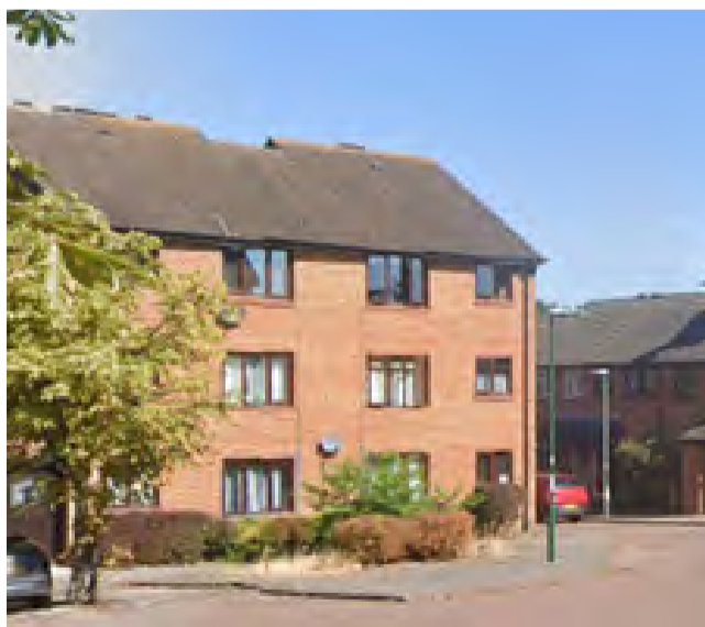
Higher density development, including flatted development, on former industrial land, can be found in Carshalton. These areas sometimes lack legibility.
