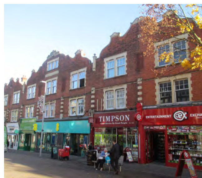
The High Street has a mix of styles and high quality shops fronts that the CA seeks to protect and enhance.
