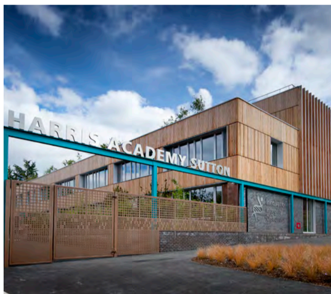
There are a number of key social infrastructure sites across the neighbourhood, including the Harris Academy Secondary School. Opened in 2018, the Passivhaus school, located on the London Cancer Hub site, has won multiple design awards.
