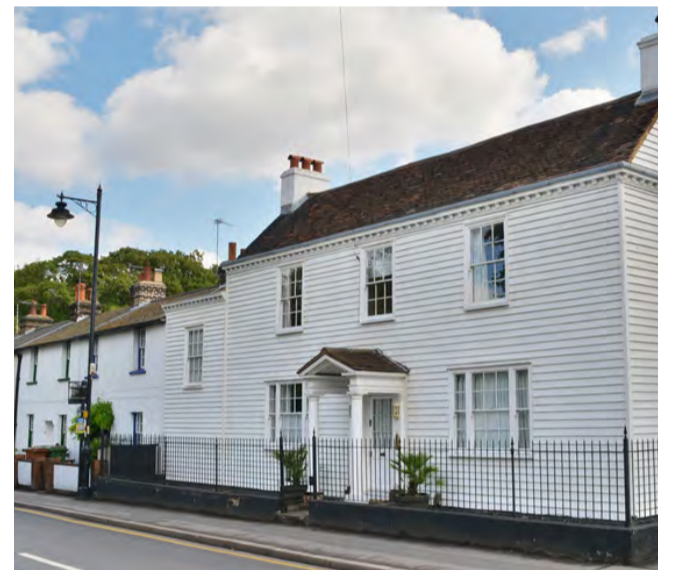
White weather-boarded houses are characteristic within parts of the Carshalton Village Conservation Area, adding to the townscape value of the neighbourhood.
