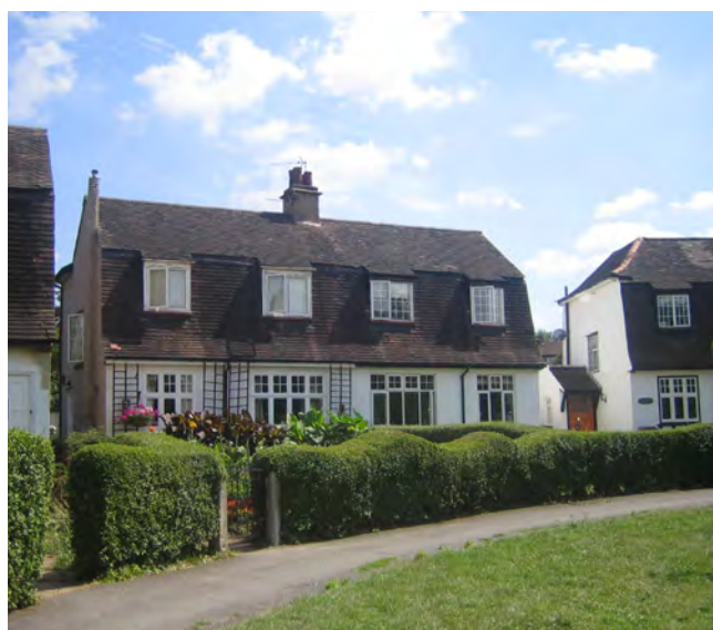
High quality low density suburban development is located immediately outside the town centre area.
