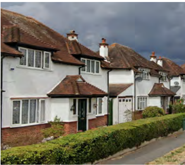
Interwar housing is the predominant housing typology surrounding the historic core of Carshalton village.
