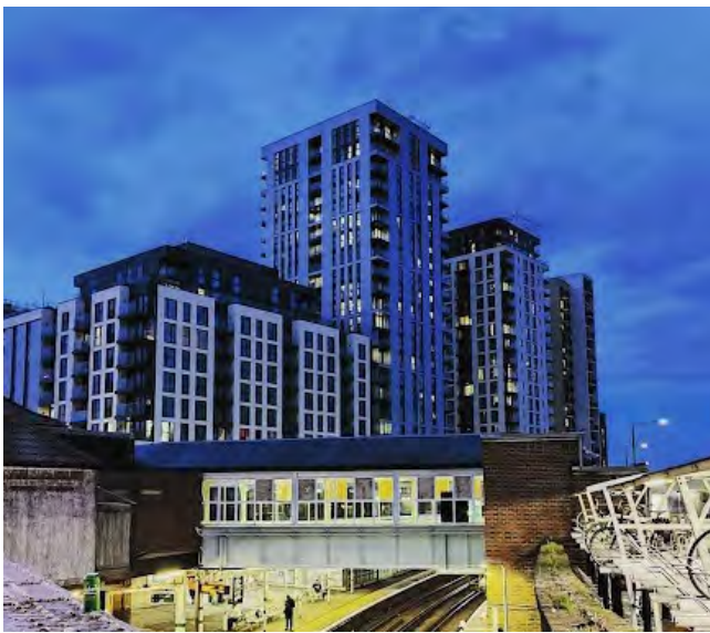
The highest density development and tallest buildings are located in Sutton Town Centre, close to Sutton station.
