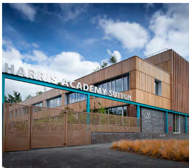
There are a number of key social infrastructure sites across the neighbourhood, including the Harris Academy Secondary School. Opened in 2018, the Passivhaus school, located on the London Cancer Hub site, has won multiple design awards.
