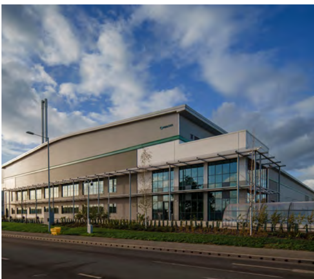
Beddington Industrial Estate is the largest industrial area in Sutton and is characterised by large box industrial units.
