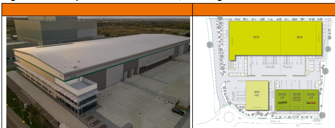
Figure 4.8 Examples of industrial units, Beddington SIL – Subarea 2
