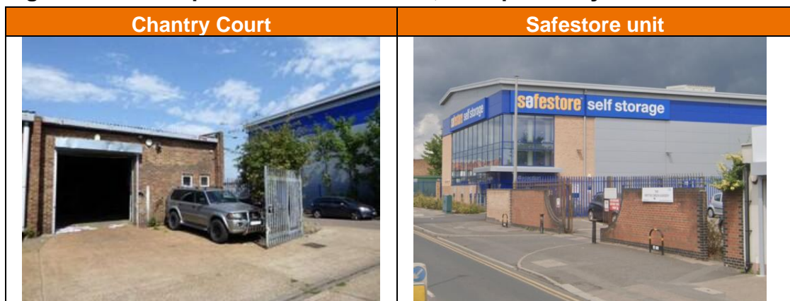
Figure 4.20 Examples of industrial units, Plumpton Way Industrial Estate
