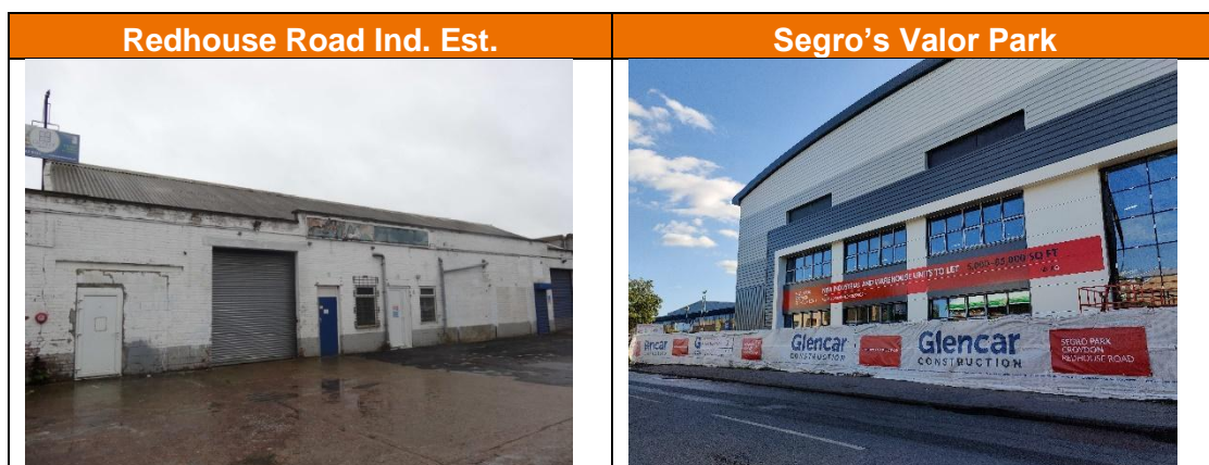
Figure 4.13 Examples of industrial units, Beddington SIL – Subarea 7
