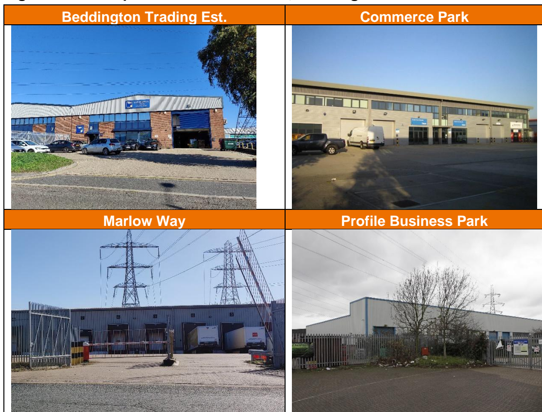
Figure 4.9 Examples of industrial units, Beddington SIL – Subarea 3
