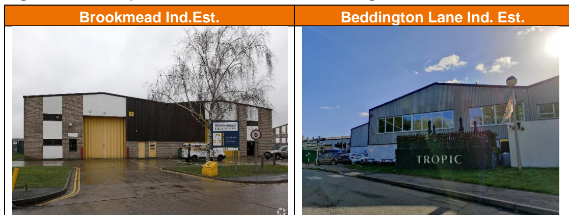
Figure 4.7 Examples of industrial units, Beddington Lane SIL – Subarea 1
