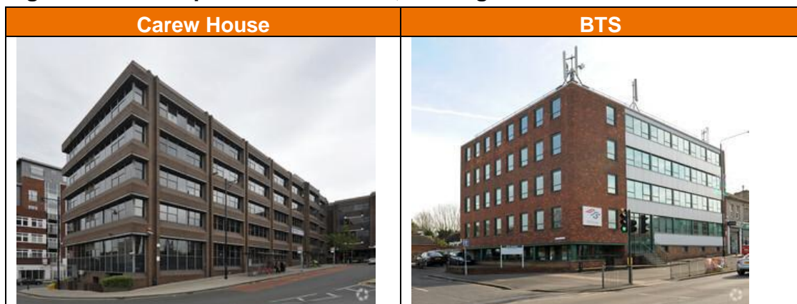
Figure 4.27 Examples of office units, Wallington
