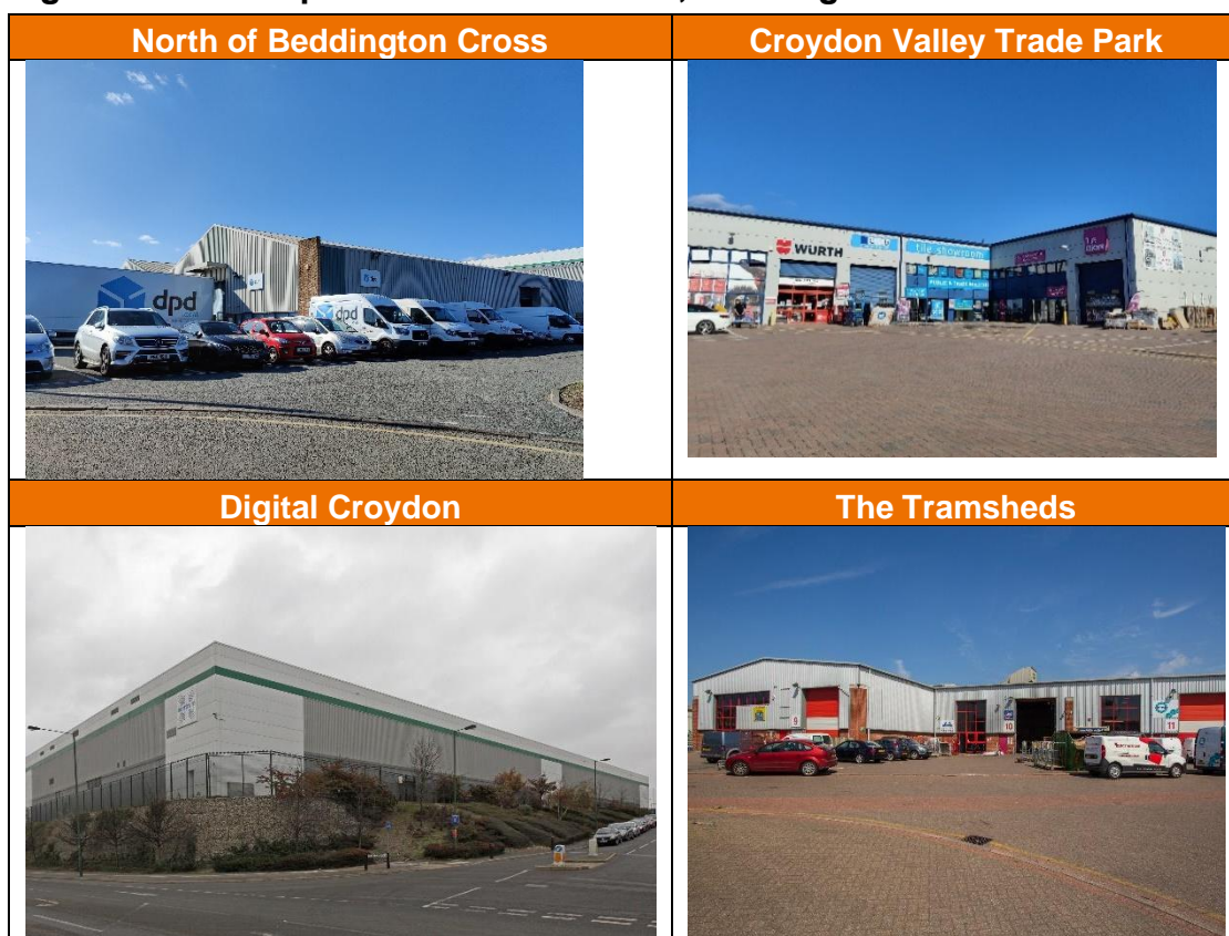
Figure 4.11 Examples of industrial units, Beddington SIL – Subarea 5
