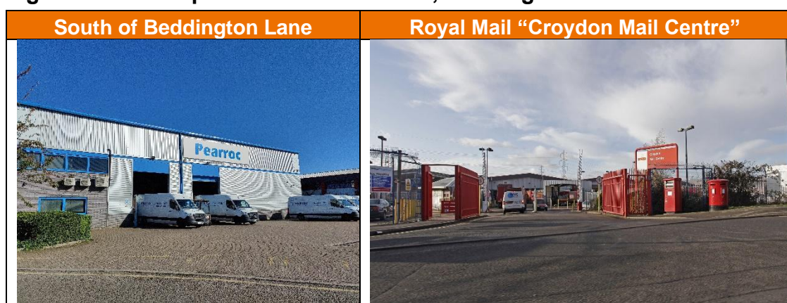
Figure 4.10 Examples of industrial units, Beddington SIL – Subarea 4
