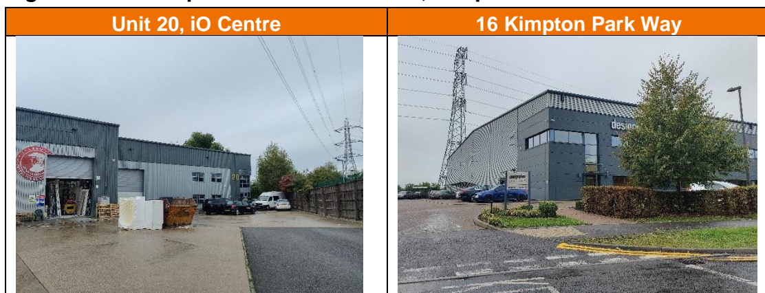
Figure 4.14 Examples of industrial units, Kimpton SIL
