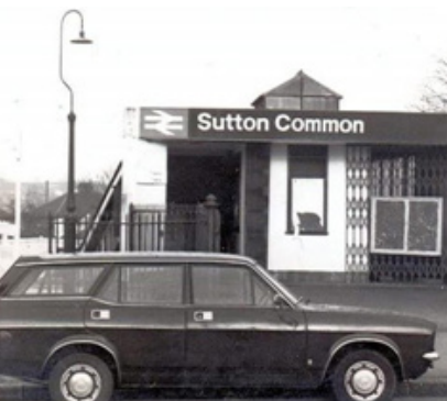
1970s station frontage, with original entrance building
