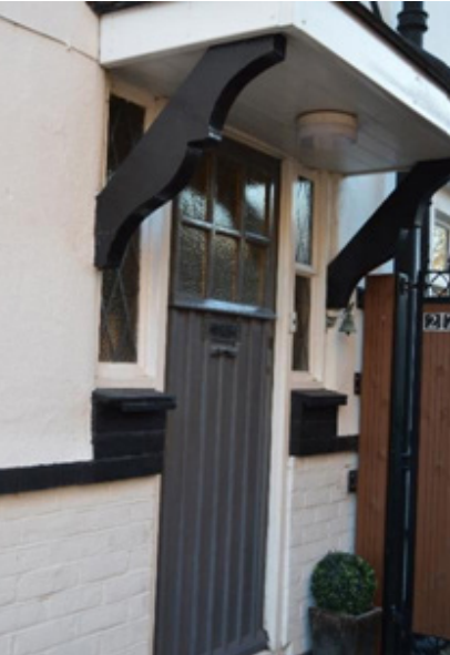
Door canopy at 26 Blenheim Road
