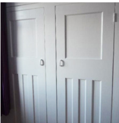
Original internal doors at 22 Blenheim Road.
