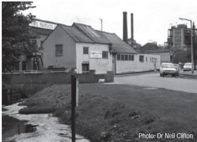
1973 Gray Gauges occupied Ansell's mill from 1967 until at least 1973. Vinyl Products Ltd. manufactured Vinyl Chloride Monomer (VCM) a liquid from which PVC is made. Land by the river in Mill Lane was a site for industry until the 1990's. British Petroleum works (in the background) was demolished in 1992 and the existing housing sites built c.1995.
