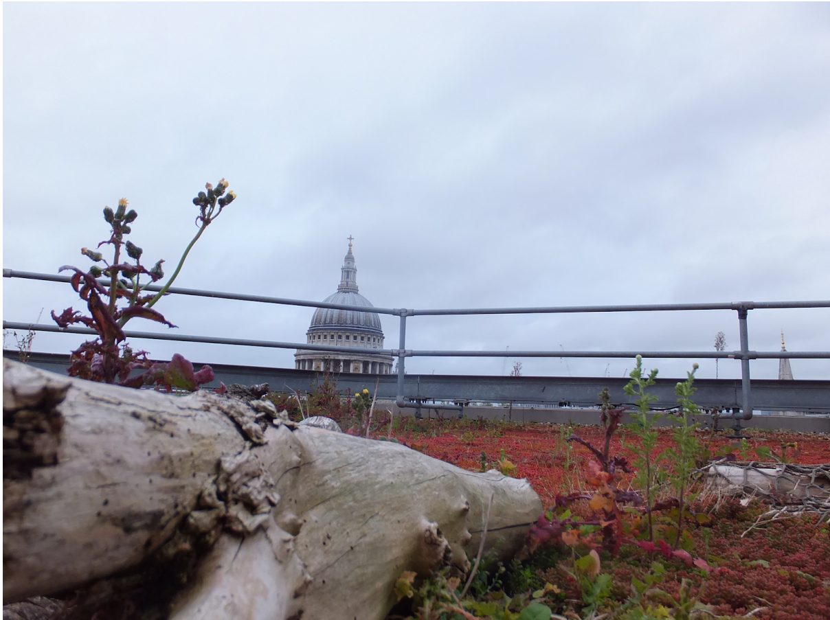
Eversheds, Wood Street - Hybrid sedum roof, with dead wood feature, looking to St. Paul's Cathedral
