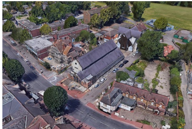
Fig 133 Google earth photography of Carshalton high street
