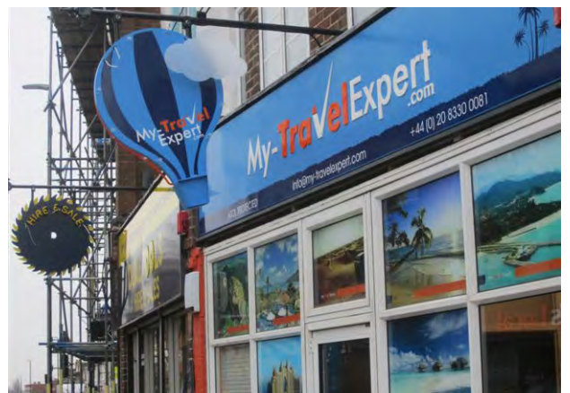
Worcester Park shop front signage improvements
