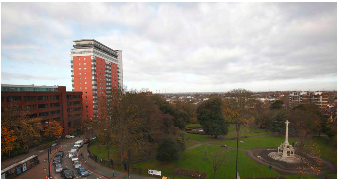
Top: view looking south up the High Street from the Gas Works site during construction Bottom: view looking north across Manor Park shows the taller buildings along Throwley Way
