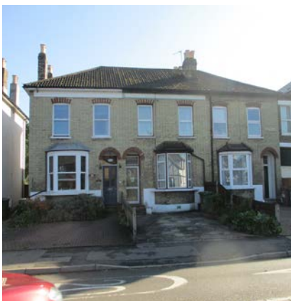
Nos 130-134 (Elm Villas) West Street
