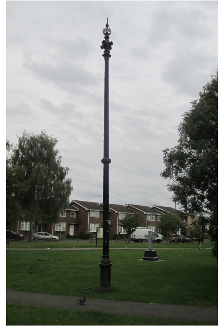
Sewer Ventilation Column
