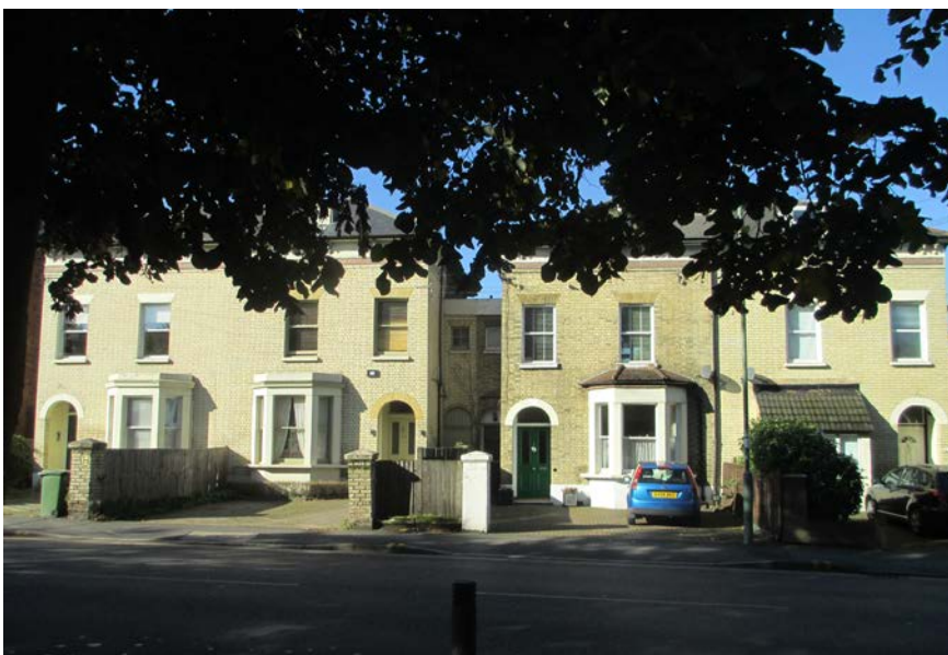
Nos 61-67 North Street
